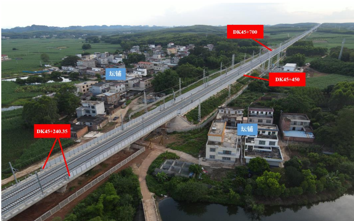
11、坛铺：坛铺特大桥 DK45+240.35~DK45+311.09 桥梁两侧声屏障；K45+311.09~DK45+450 路基右侧、K45+311.09~DK45+700 路基左侧高声屏障
