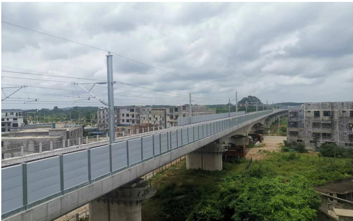
8、光明南路居民点：吴圩特大桥DK23+991.45~DK24+300.8桥梁右侧、DK24+155.25~DK24+260桥梁左侧声屏障
