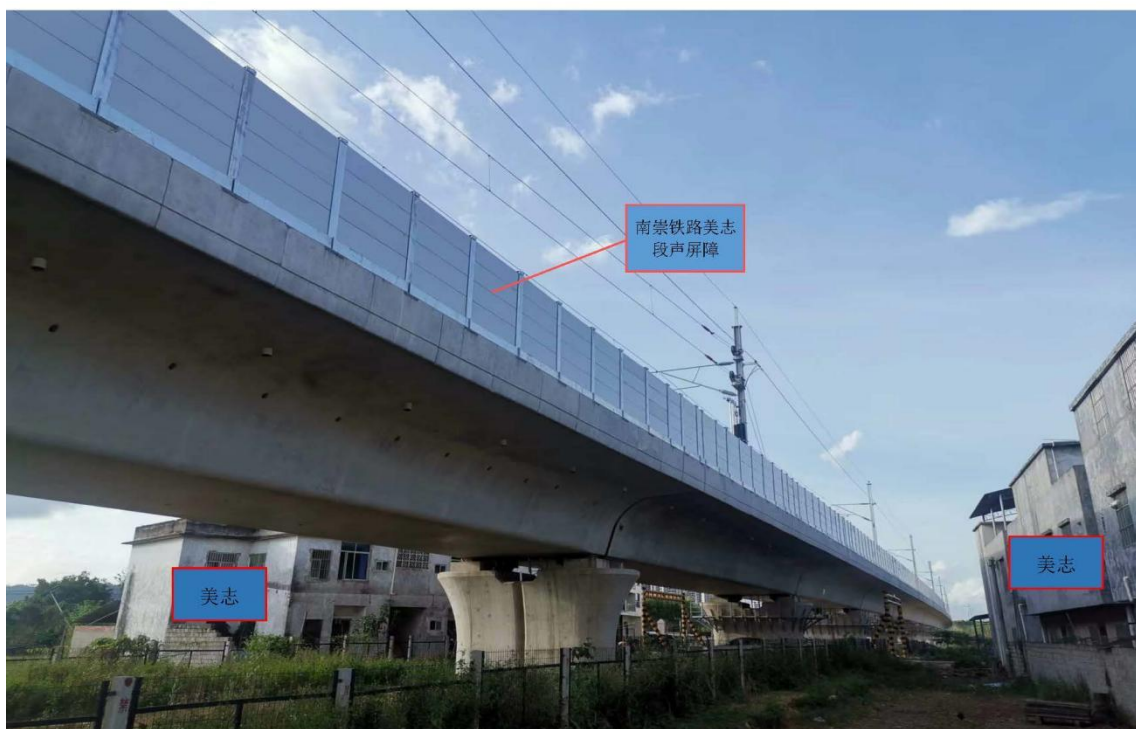
6、美志：吴圩特大桥DK22+256.23~DK22+616.37桥梁左侧声屏障
